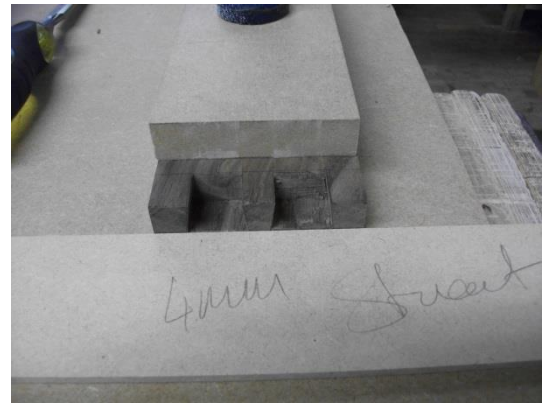
Event no. 22 – Using gauge to cut out lapped sockets
